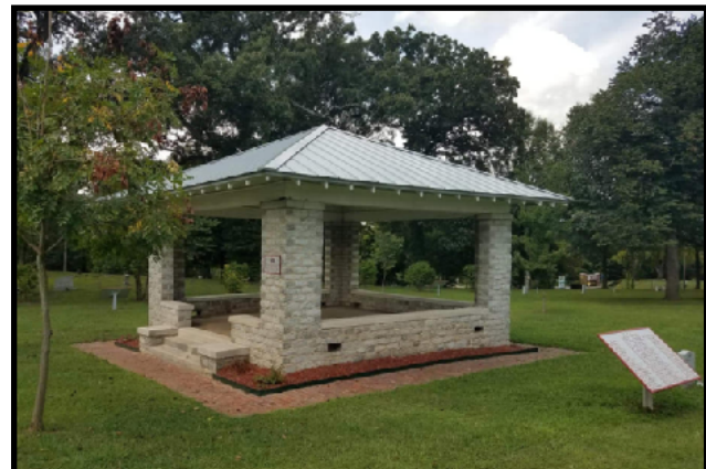
Lt. Commander Billy Walker of N. B. Forrest Camp #3 in Chattanooga presents photos of the newly completed roof on the pavilion in the Chattanooga Confederate Cemetery.
